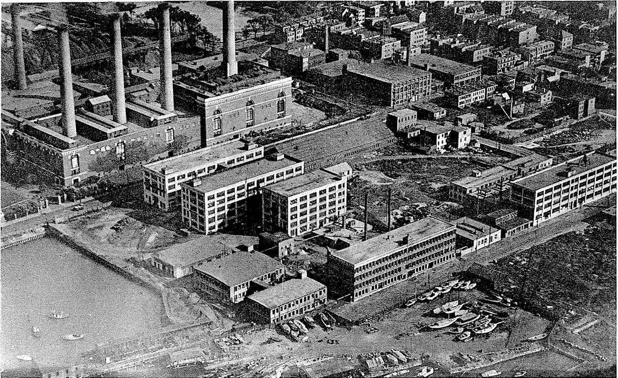
KING TERMINAL BUILDINGS, SOUTH BOSTON, MASS. / 250.000.
