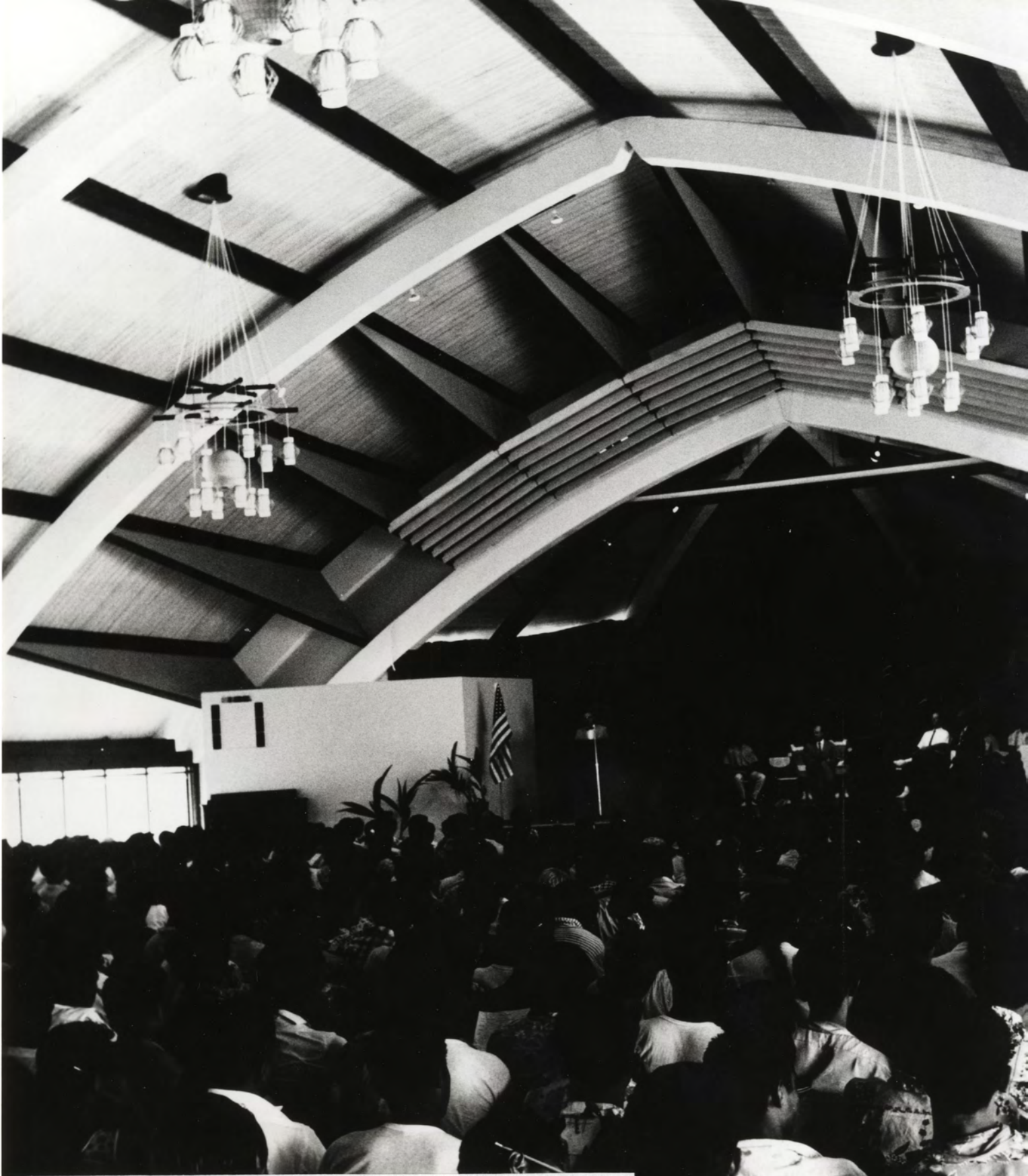
AMERICAN SAMOA CIVIC AUDITORIUM Showing three-hinge arch See photo exhibit for finished product.
