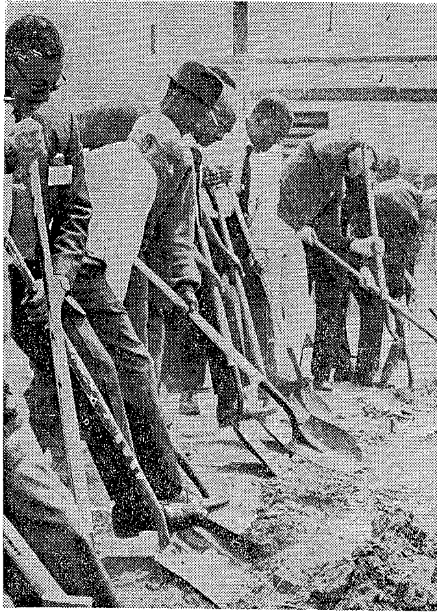
DIG, BABY, DIG —Watts community leaders and friends pitch in with shovels to dig trenches for the foundation of a new Community Art Center.
