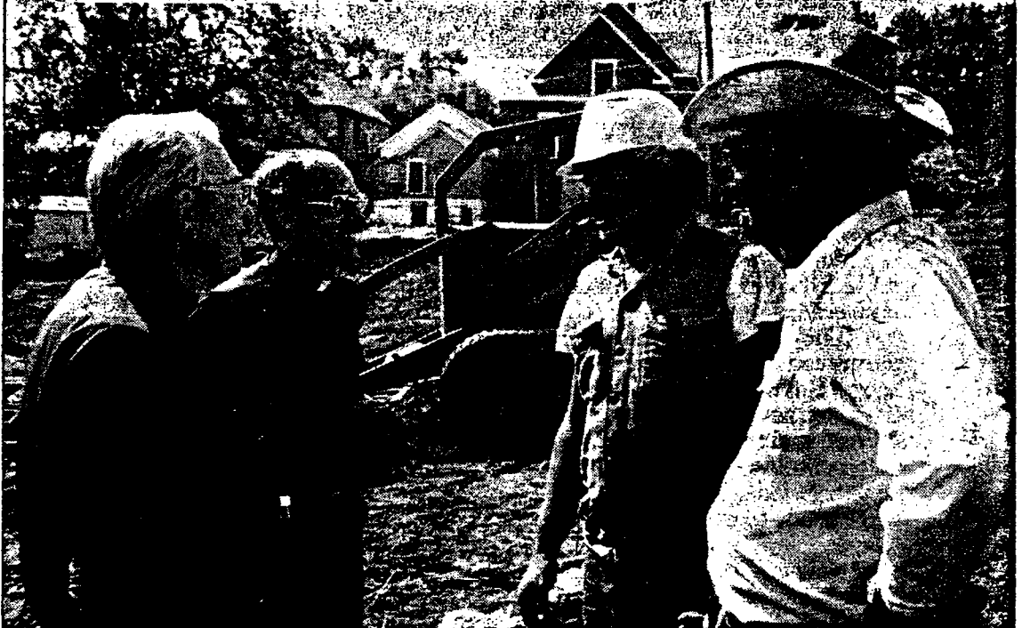
Awaiting site clearance . . . l-r Rathers Hupp and Gilg, workers Walter Lowe and Wes Taylor.
