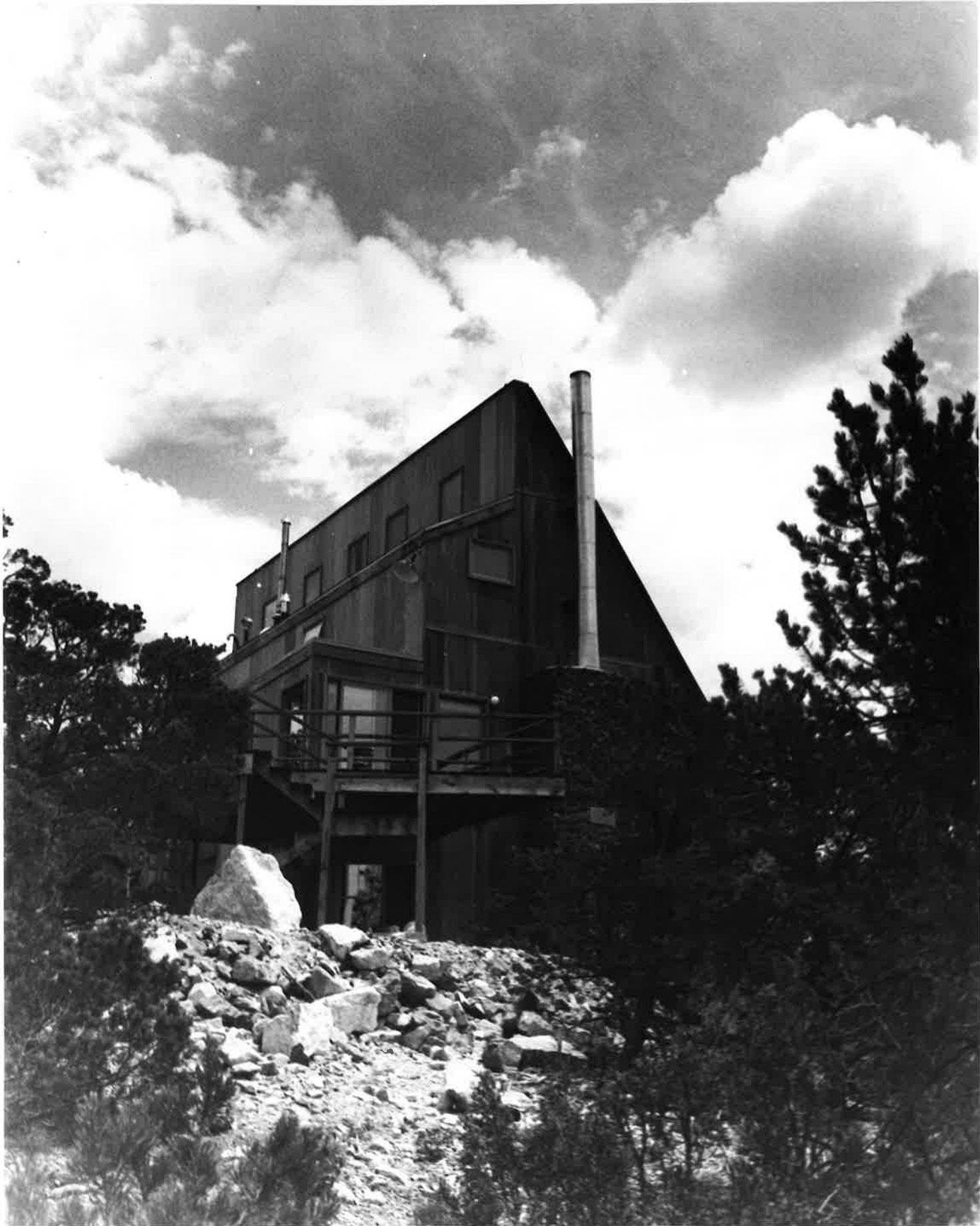
ARCHITECT OF RECORD DON P. SCHLEGEL DESIGNER DON P. SCHLEGEL PROJECT FRANK ZANNER ACTIVE SOLAR HOUSE DATE 1976 AUTHORSHIP: Solely Responsible for Design DON P. SCHLEGEL
