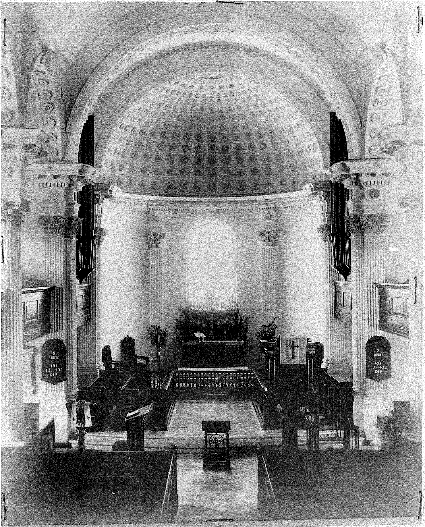
New Choir and Chancel added to St Philip's Church Charleston, S.C. 1920. (Stained Glass window not installed at time of photograph) Simons and Lapham, Architects, Charleston, S.C.
