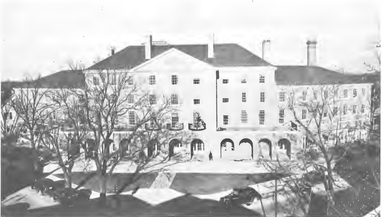
Tidewater Inn, Easton, Maryland
