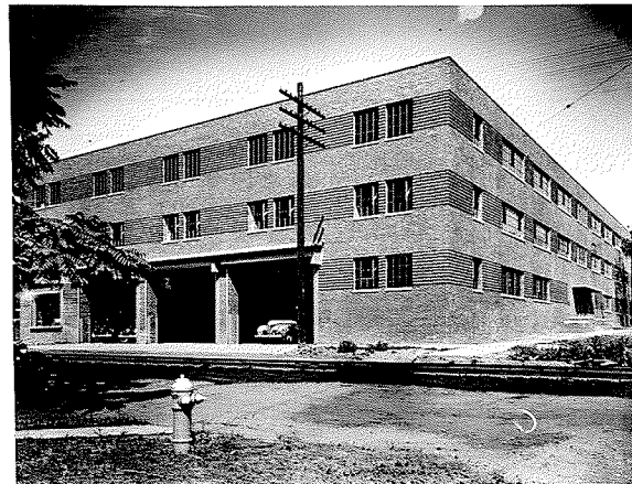
SUTLIFF & CASE WAREHOUSE 80' x 125' FRONT & SIDE ELEVATION SIZE 171'-3" x 128'-0" COST $125,000
