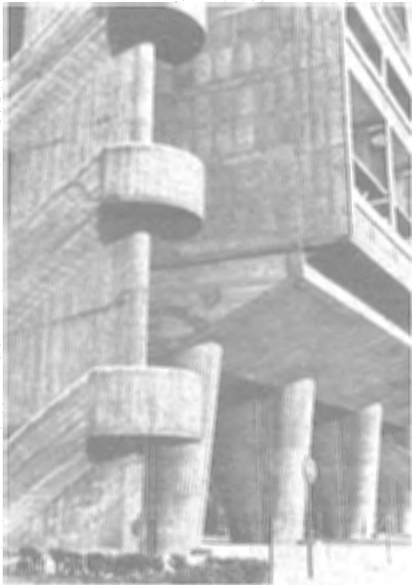
Ground floor of an Apartment House by Le Corbusier. Unfinished concrete
