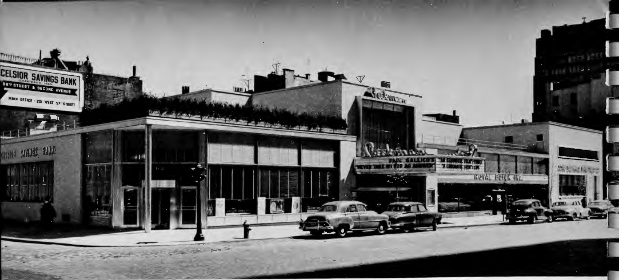
NEW YORK LIFE INSURANCE CO., COMMERCIAL BLOCK WITH THEATRE AND BRANCH BANKS
