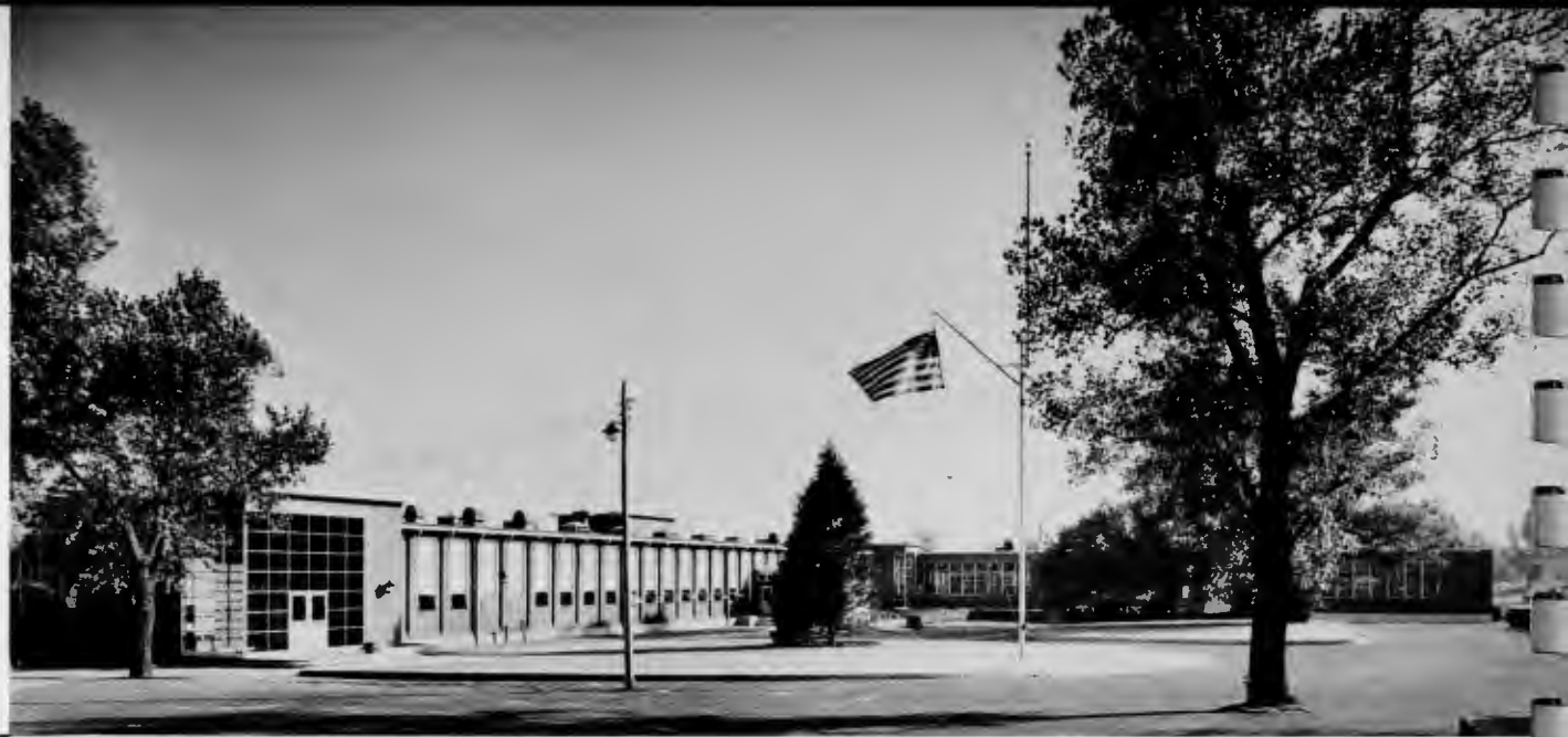
BECTON, DICKINSON & CO. SHIPPING BUILDING AND ONE OF PRODUCTION BUILDINGS
