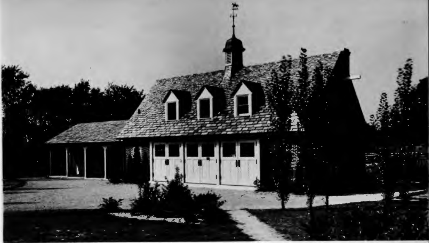
GARAGE AND STABLE
