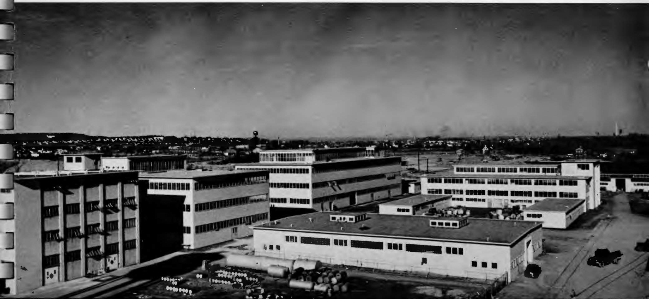
GENERAL VIEW OF PLANT BUILDINGS
