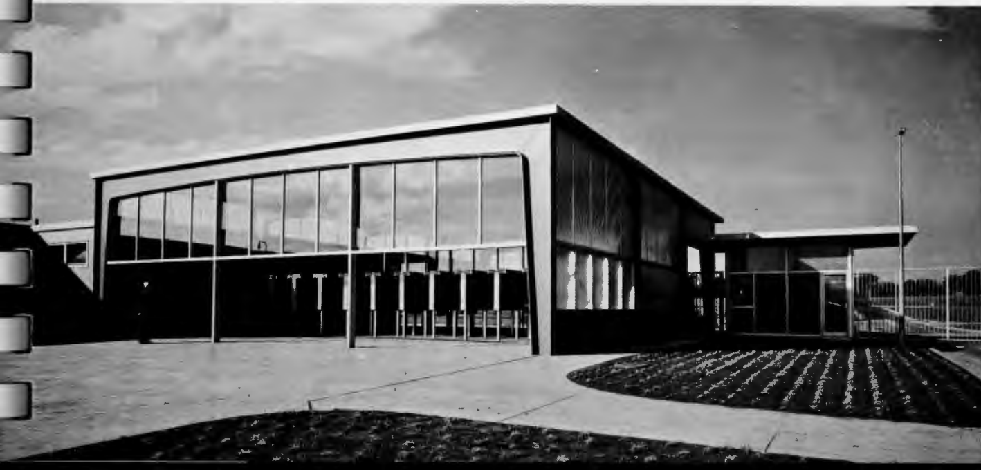
PLANT SAFETY AND EMPLOYMENT BUILDING
