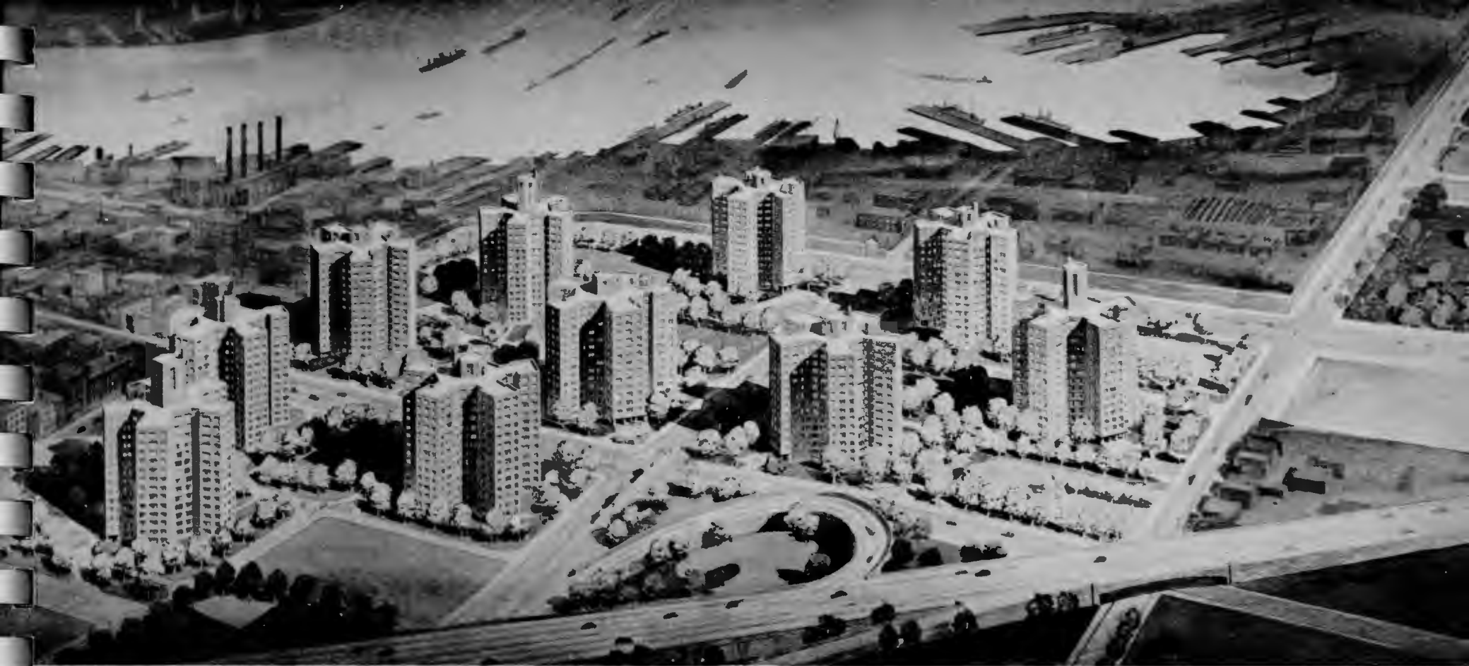
NEW YORK CITY HOUSING AUTHORITY, FARRAGUT HOUSES, BROOKLYN, N. Y.
