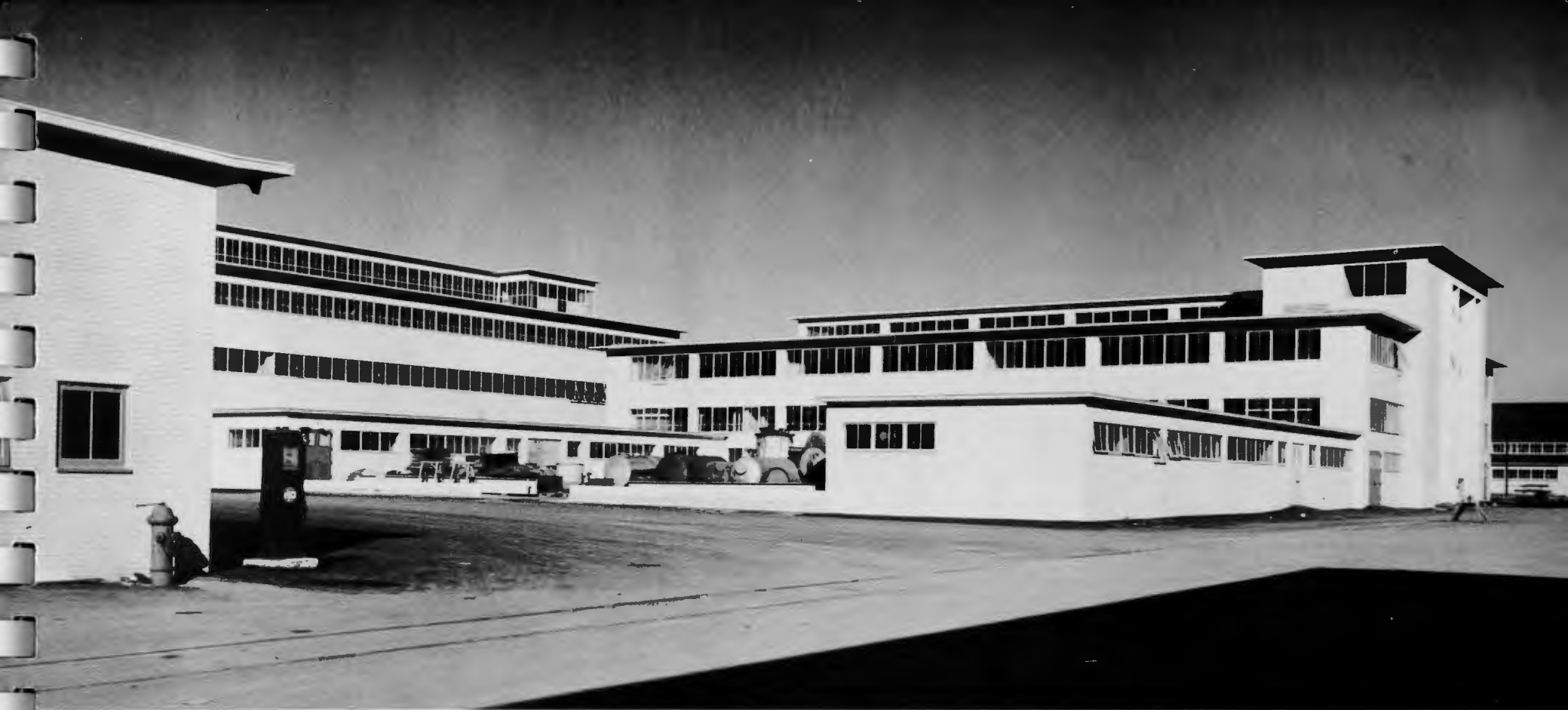
PRODUCTION BUILDING AND SHOP
