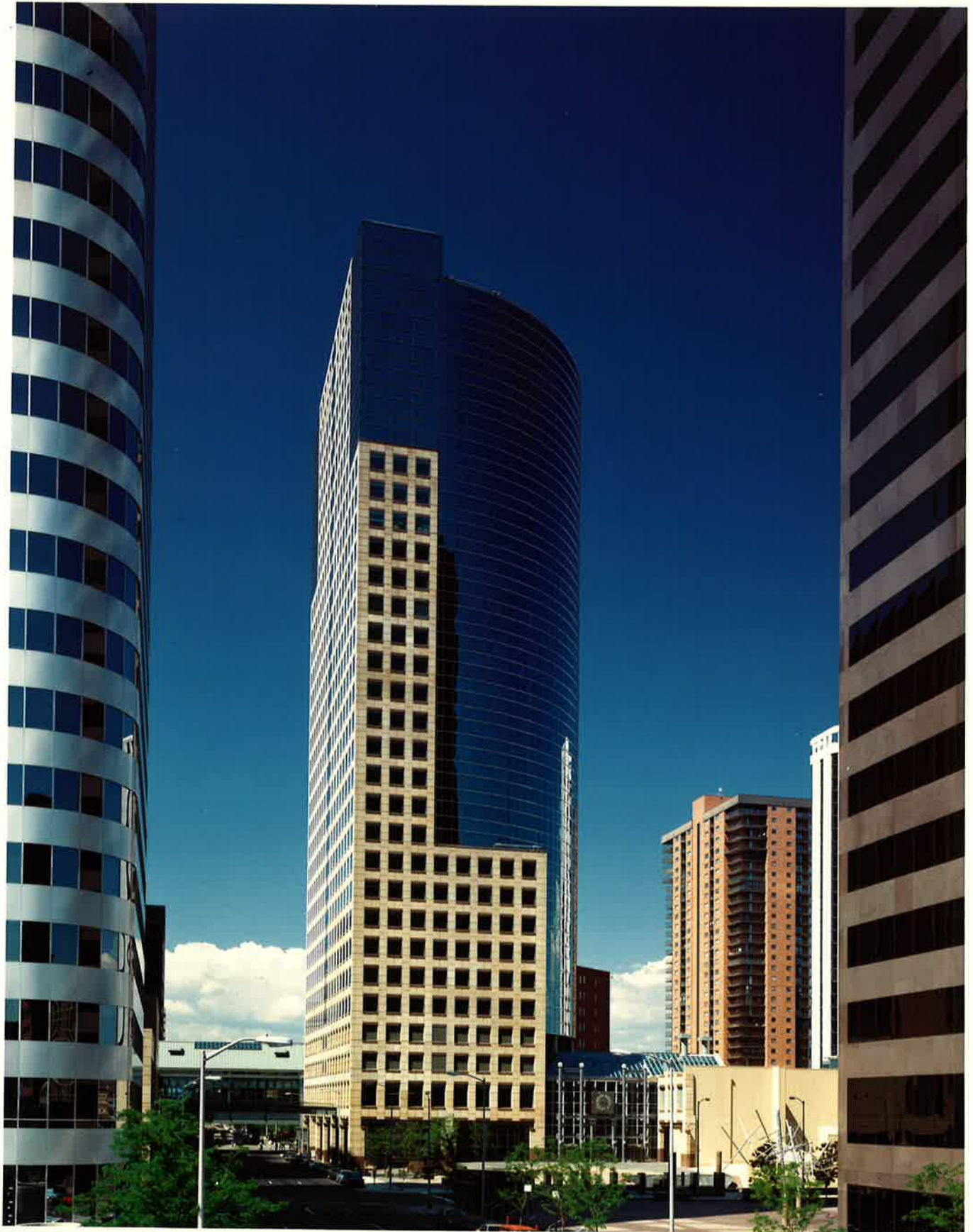
ARCHITECT OF RECORD KOHN PEDERSEN FOX ASSOCIATES PC DESIGNER PROJECT TABOR CENTER DATE 1985 AUTHORSHIP: Largely Responsible for Design and Partner in Charge
