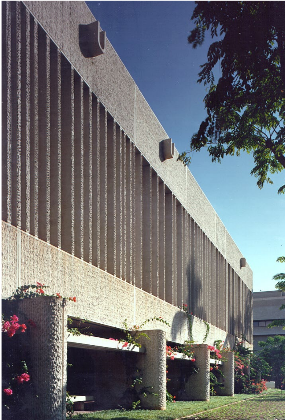
Arcade Around Building
