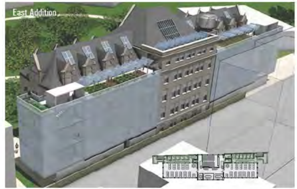
Above View from the Southeast showing proposed additions to original circa 1908 building and green roof areas
