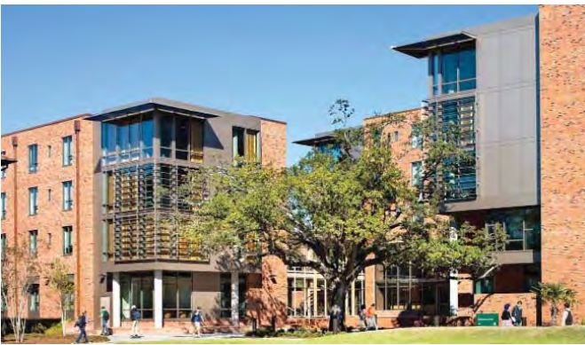
21 Weatherhead Hall. 2011. Hanbury Evans Wright Vlattas + Company / John C. Williams Architects
