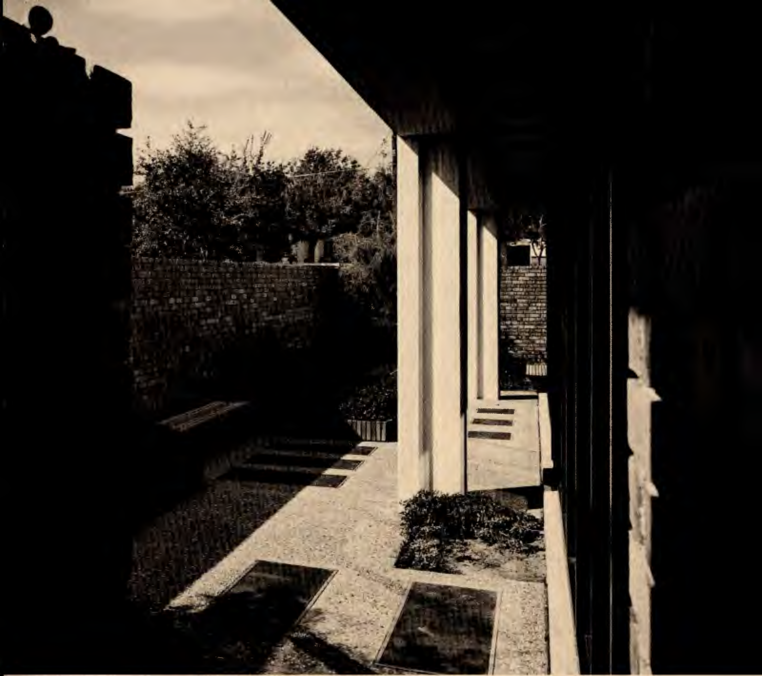
Corporate Headquarters & Research Facilities, Dixico Inc., Dallas
