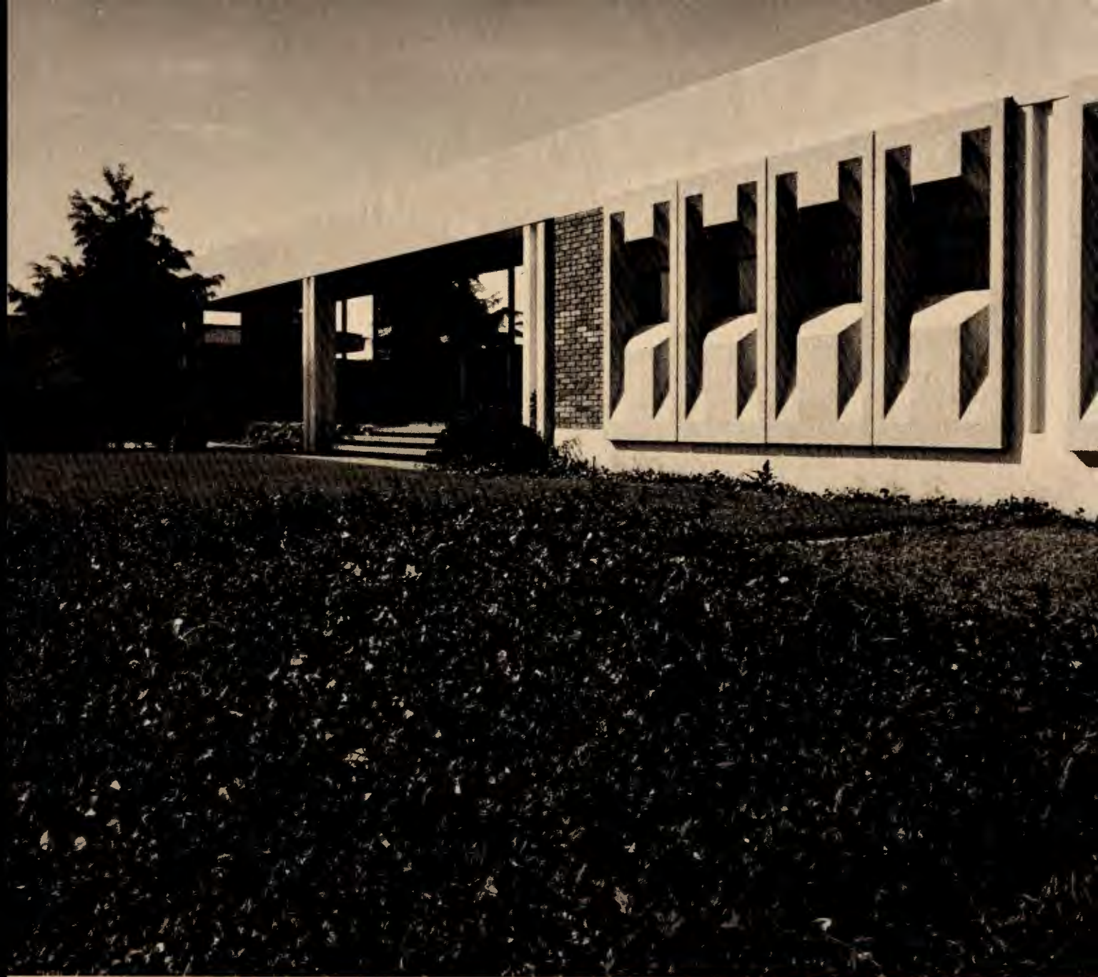
Corporate Headquarters & Research Facilities, Dixico Inc., Dallas
