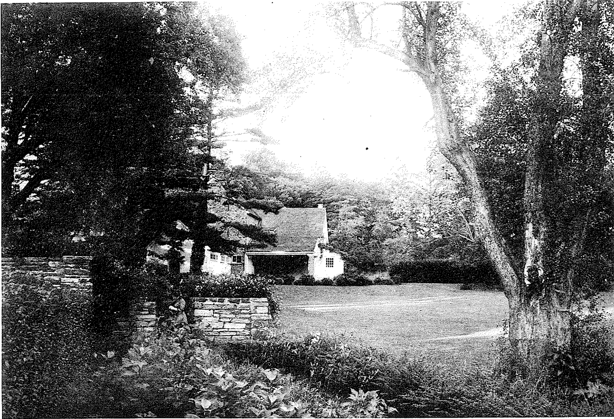
THE HOME OF FRANK MILES DAY AT MT. AIRY NEAR PHILADELPHIA
