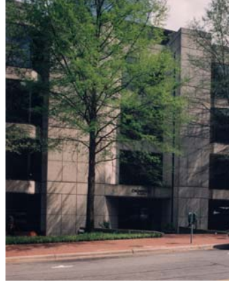
One Spring Building
