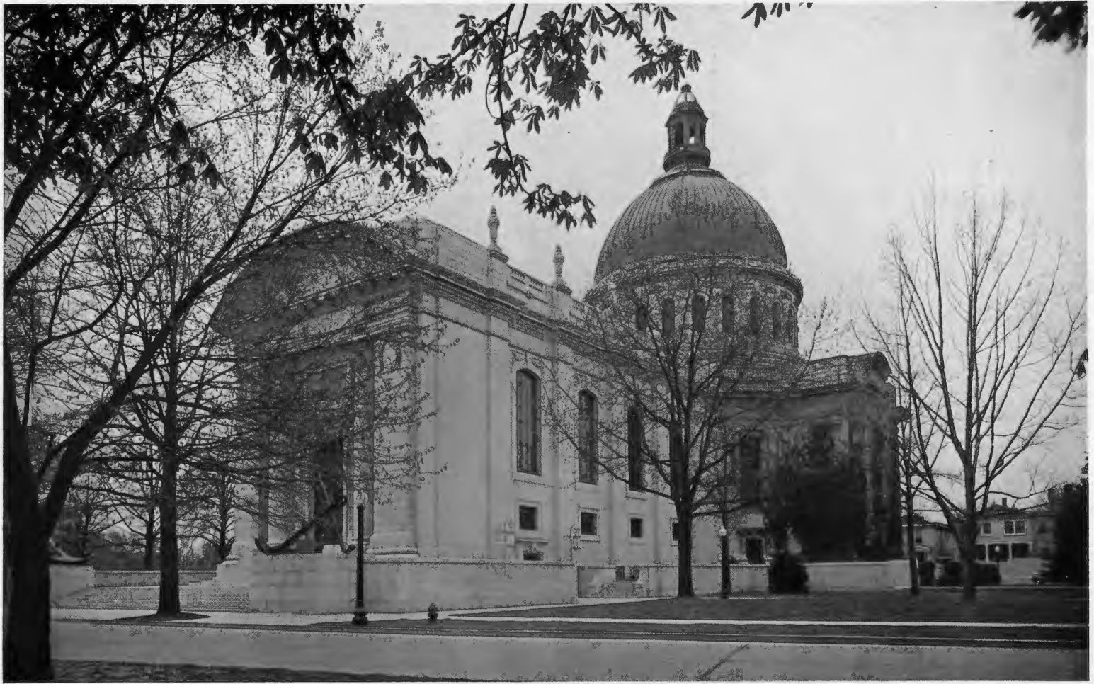
(Above) Chapel, U. S. Naval Academy, Annapolis, Maryland. Architect of original building: Ernest Flagg. Architect of Extension to the Nave: Paul P. Cret.
