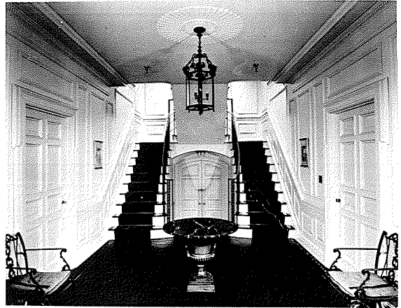
LOBBY INTERIOR, OFFICE BUILDING, NORWALK, CONN. 60,000 Sq. Ft., $300,000. EDWARDS & COMPANY.
