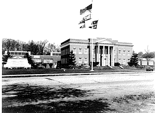
FRONT VIEW, OFFICE & FACTORY, NORWALK, CONN. 60,000 Sq. Ft. $300,000 EDWARDS & COMPANY
