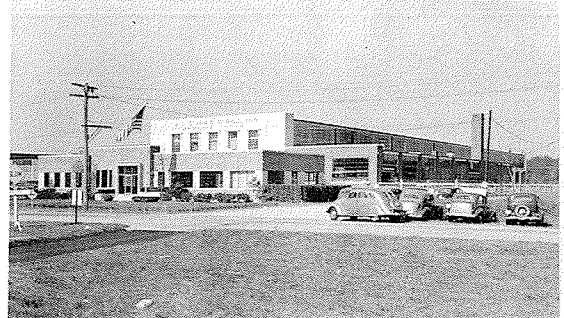
PERSPECTIVE VIEW, OFFICE & SHOP, FAIRFIELD, CONN. 20,000 Sq. Ft. $235,000 J.L. LUCAS & SON, INC.
