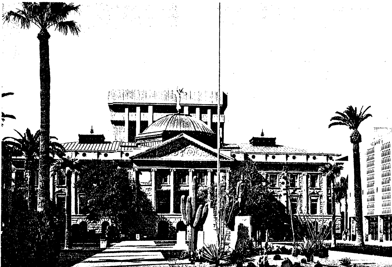
The Restored Arizona Capitol Museum, now partially framed by recent capitol addition. copper roofing: Goettl Brothers Metal Products, Inc., Phoenix
