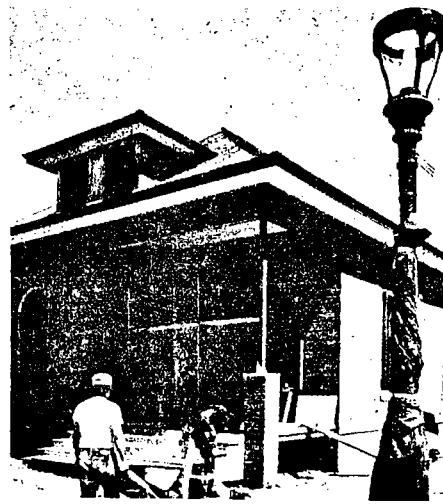
Teater House in Heritage Square, a typical turn-of-the-century Phoenix home, is costing $100 per square foot to restore. Because the bricks had cracked with wear, workmen had to turn them inside out.
