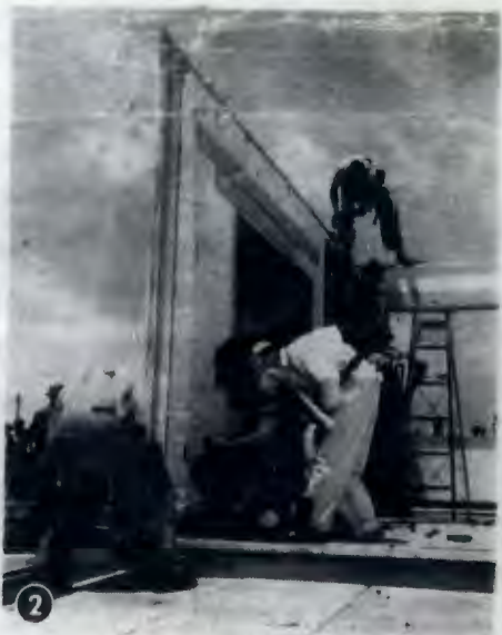
With one wall already up, workmen tighten its connections to frame and get ready for next one.
