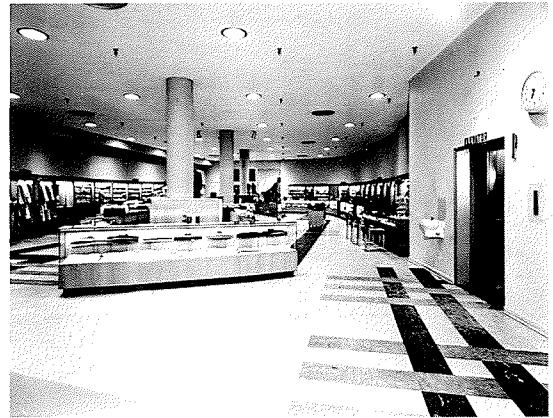
FIRST FLOOR LOOKING EAST SIEGEL'S, SAN ANTONIO, TEXAS 24,000 sq. ft. $200,000 MR. SYLVAN LANG, et al
