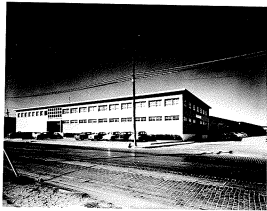
EAST ELEVATION PERRY SHANKLE CO. SAN ANTONIO, TEXAS 104,000 sq. ft. $400,000 PERRY SHANKLE CO. SAN ANTONIO, TEXAS
