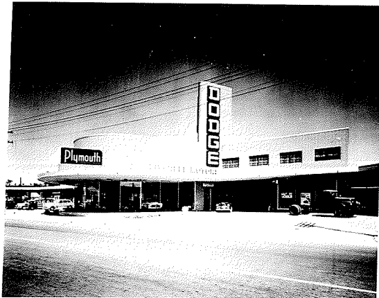
EST ELEVATION R. MITCHELL MOTORS, SAN ANTONIO, TEXAS 0,000 sq. ft. 350,000 IR. OR. MITCHELL, SAN ANTONIO, TEXAS
