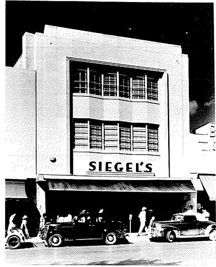
EAST (front) ELEVATION SIEGEL'S, SAN ANTONIO, TEXAS 24,000 sq. ft. $200,000 MR. SYLVAN LANG, et al
