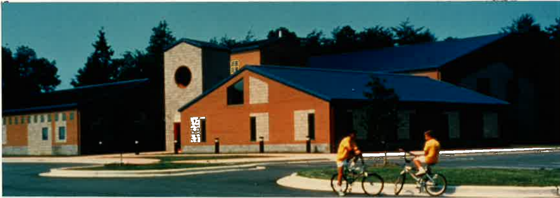
From the outside, the Center looks to be a cluster of patched up gable roof structures, like many others on the base.
