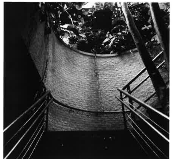
Brick-size, split-face CMU, colored to the shade of the forest floor, forms the curved surfaces of the sink hole.
