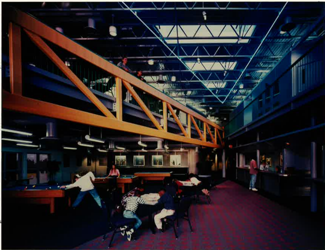
A long truss provides a columnless gaming space in what was the old gym.
