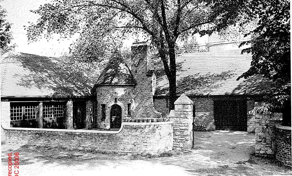
PERRYSBURG VILLAGE SERVICE BUILDING PERRYSBURG, OHIO
