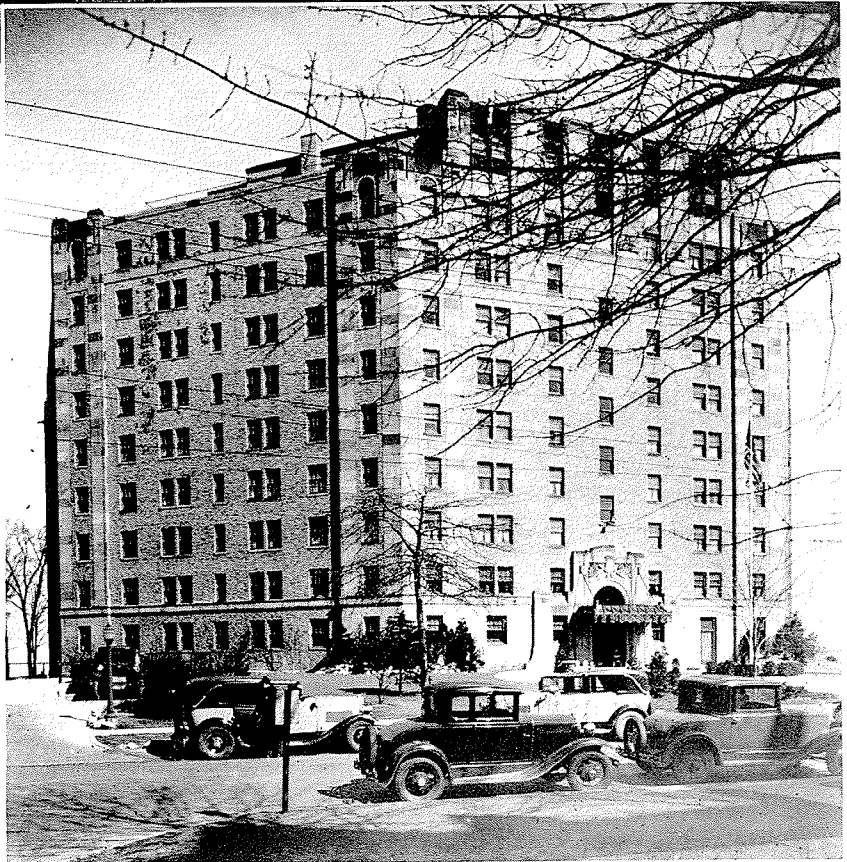
Edgewater Drive Facade
