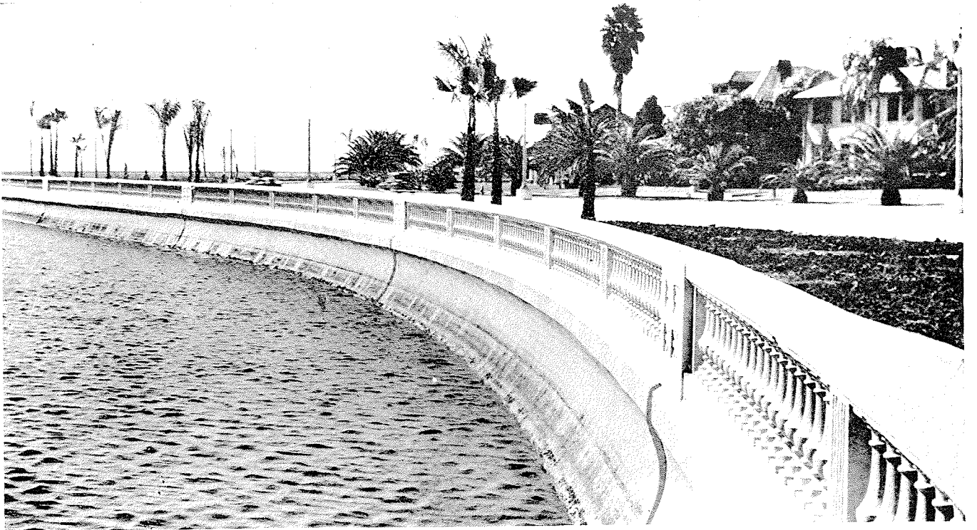
Bayshore Seawall at curve
