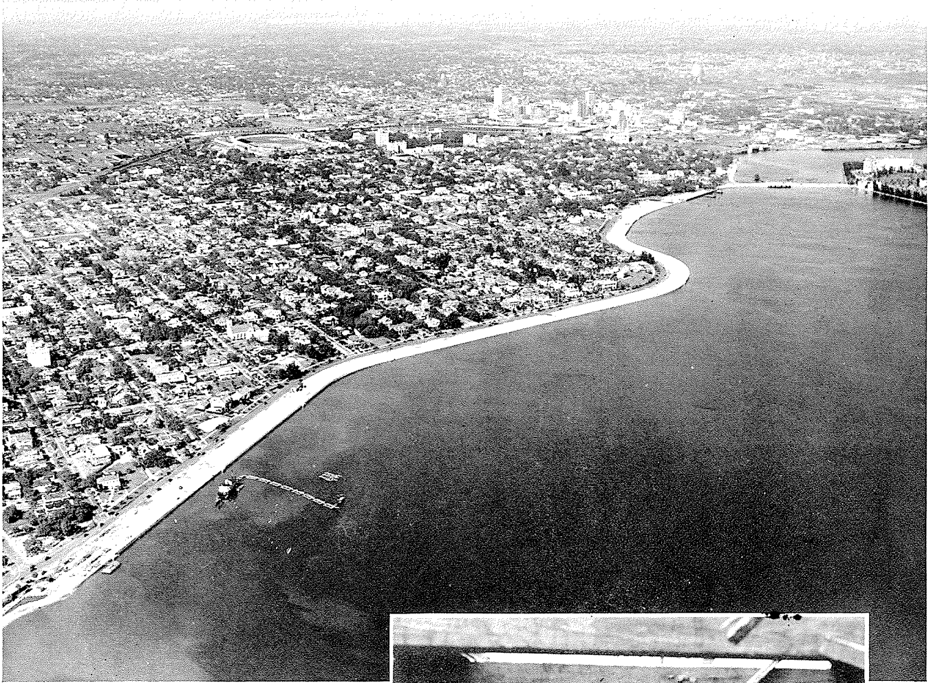
Bayshore Seawall and Bayshore Drive Tampa, Florida (Under Construction)
