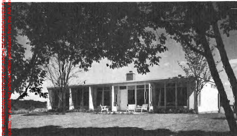
GREEN PRE-FABRICATED HOUSE MCKFORD, ILLINOIS, 1945
