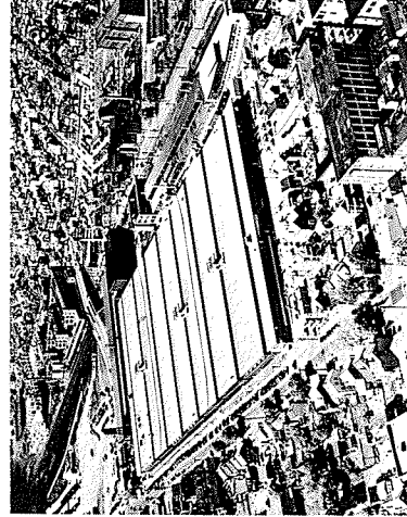
AERIAL VIEW ENGINE ASSEMBLY BUILDING WRIGHT AERONAUTICAL CORPORATION PATERSON, NEW JERSEY 515,600 SQ. FT. COST $1,416,178.00
