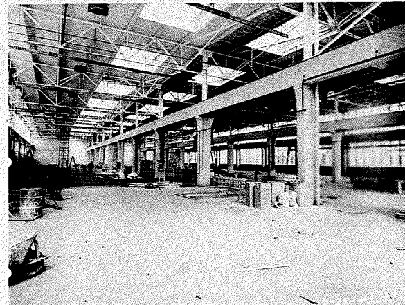
• INTERIOR VIEW - MACHINE SHOP TO THE RIGHT - DIESEL DIVISION - G.M.C.
