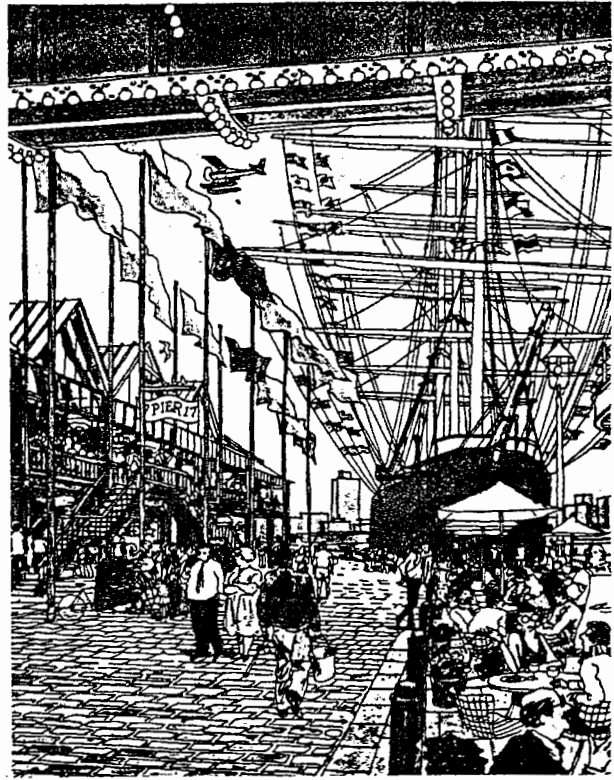
Looking east toward the Pier Pavilion.
