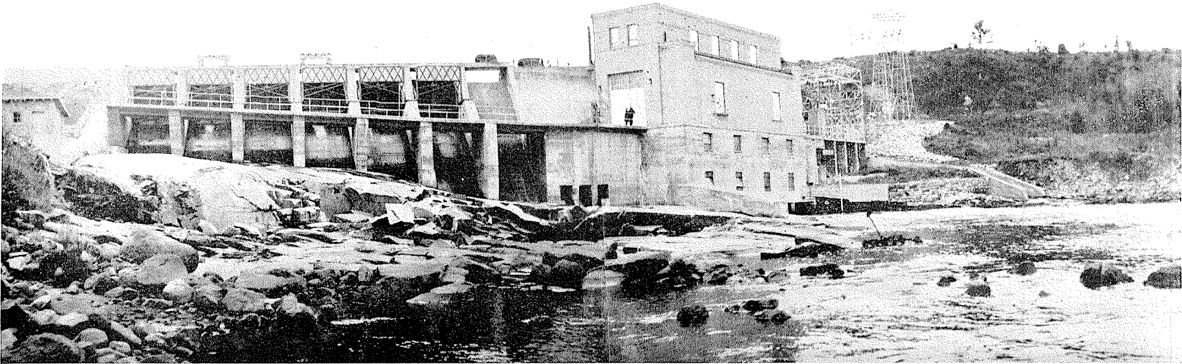
Johnson's Falls hydroelectric plant on Peshtigo River near Crivitz, Wisconsin, Wisconsin Public Service Corporation
