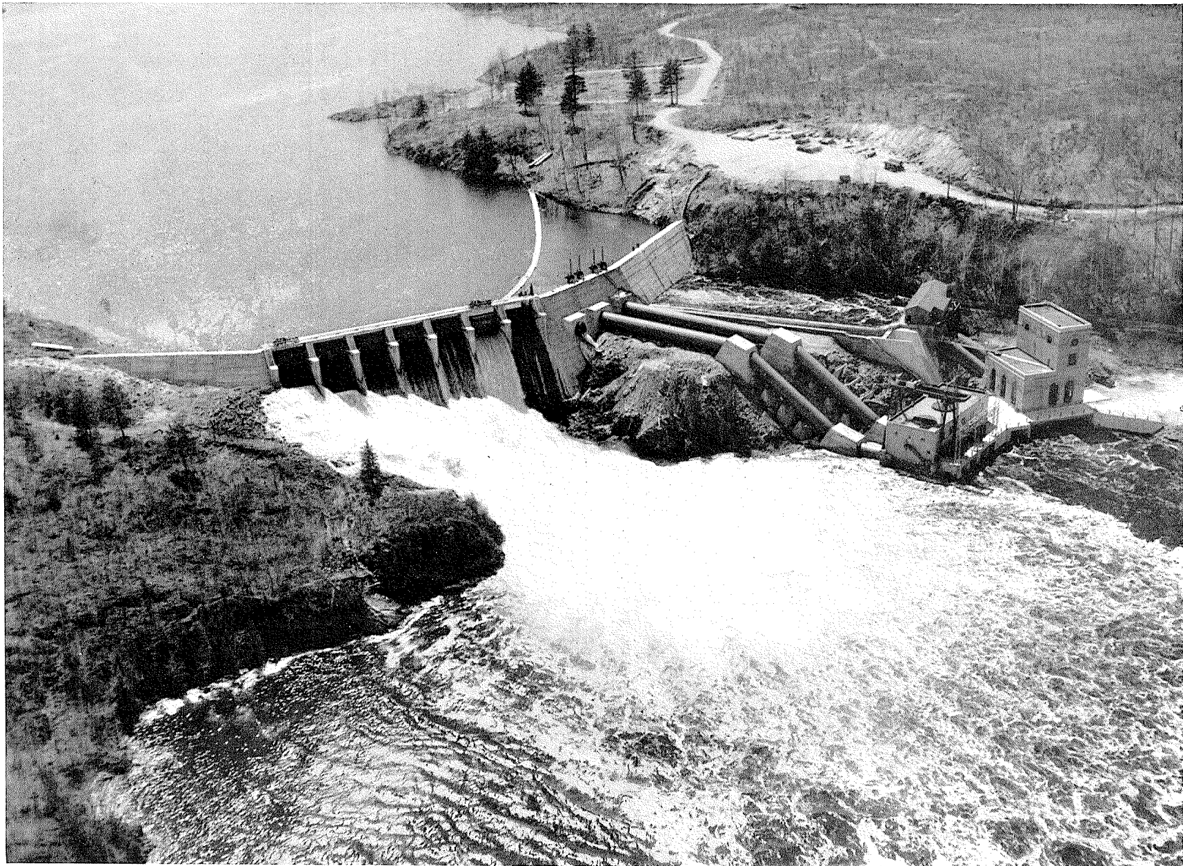
Aerial view of Big Quinnesec Falls hydroelectric plant on Menominee River near Iron Mountain, Michigan . Wisconsin-Michigan Power Company. Plant in foreground, completed in 1949, operates under 92' head; plant in background, completed in 1913, operates under 61' head.
