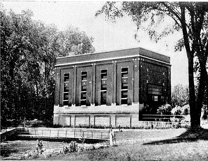
Rockton hydroelectric plant on Rock River at Rockton, Illinois, Wisconsin Power and Light Company.
