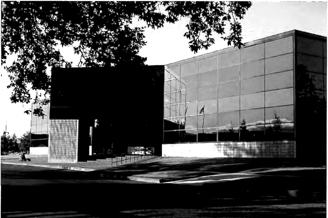
Digital Equipment Corporation Santa Clara, California
