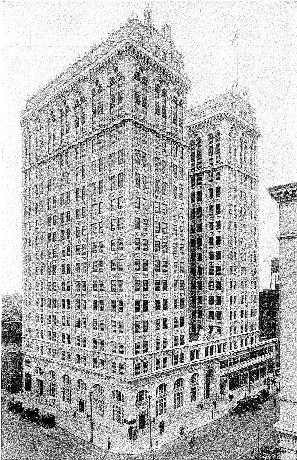
The fine seventeen-story office building owned by the Jefferson Standard Life Insurance Company, of Greensboro, North Carolina.
