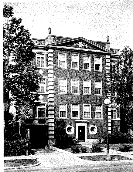
FRONT ELEVATION APARTMENT BLDG FOR MR CHAS KUSEL 50. SHORE DRIVE, CHICAGO — 60'-0" X 100'-0" — COST 75,000
