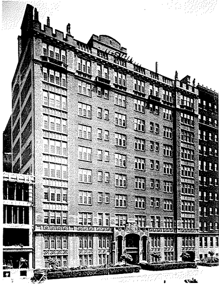
FRONT ELEVATION APARTMENT BLDG FOR MR HUGH Mc LENNAN 220 E. WALTON, CHICAGO — 100'-0" X 104'-0" — COST 600,000
