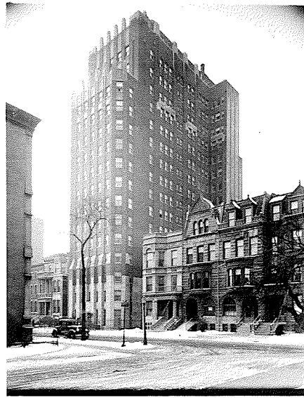
FRONT ELEVATION APARTMENT HOTEL FOR MR FRED BRONS 1220 NO. STATE, CHICAGO — 80'-0" X 150'-0" — COST 900,000
