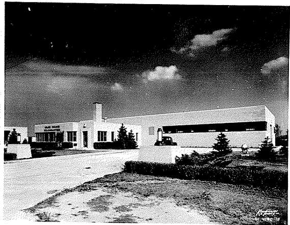
WEST ELEVATION POLICE HQTS BLDG FOR STATE OF ILL. BLUE ISLAND ILLINOIS 16,000 SQ. FT. COST 45,000
