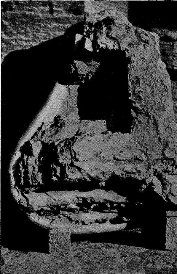
FIGURE 10A.—FRAGMENT OF GROINED VAULTING
