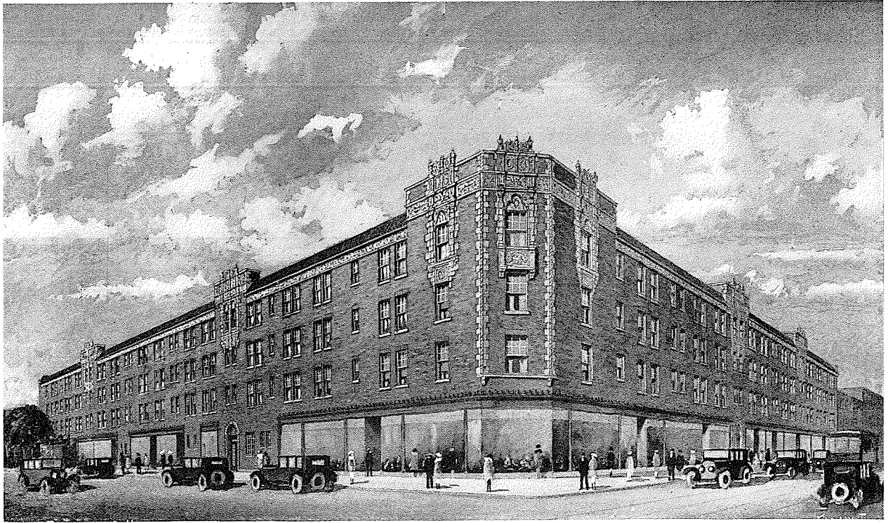
Drawing of Hotel S. E. Cor. Milwaukee and Diversey (Under Construction)
