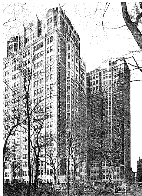
LAKE VIEW APARTMENT BUILDING 2440 Lake View Avenue
