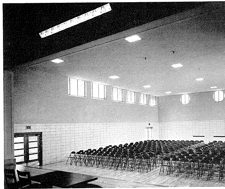
A wainscot of National Fireproofing 8 by 16-in. tile rims the au
