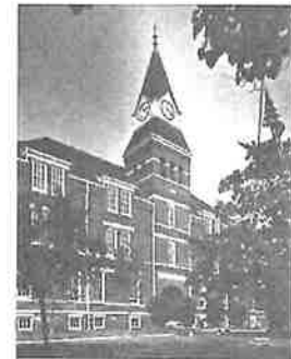
Fountain Hall Restoration, 1981 Morris Brown College Campus
