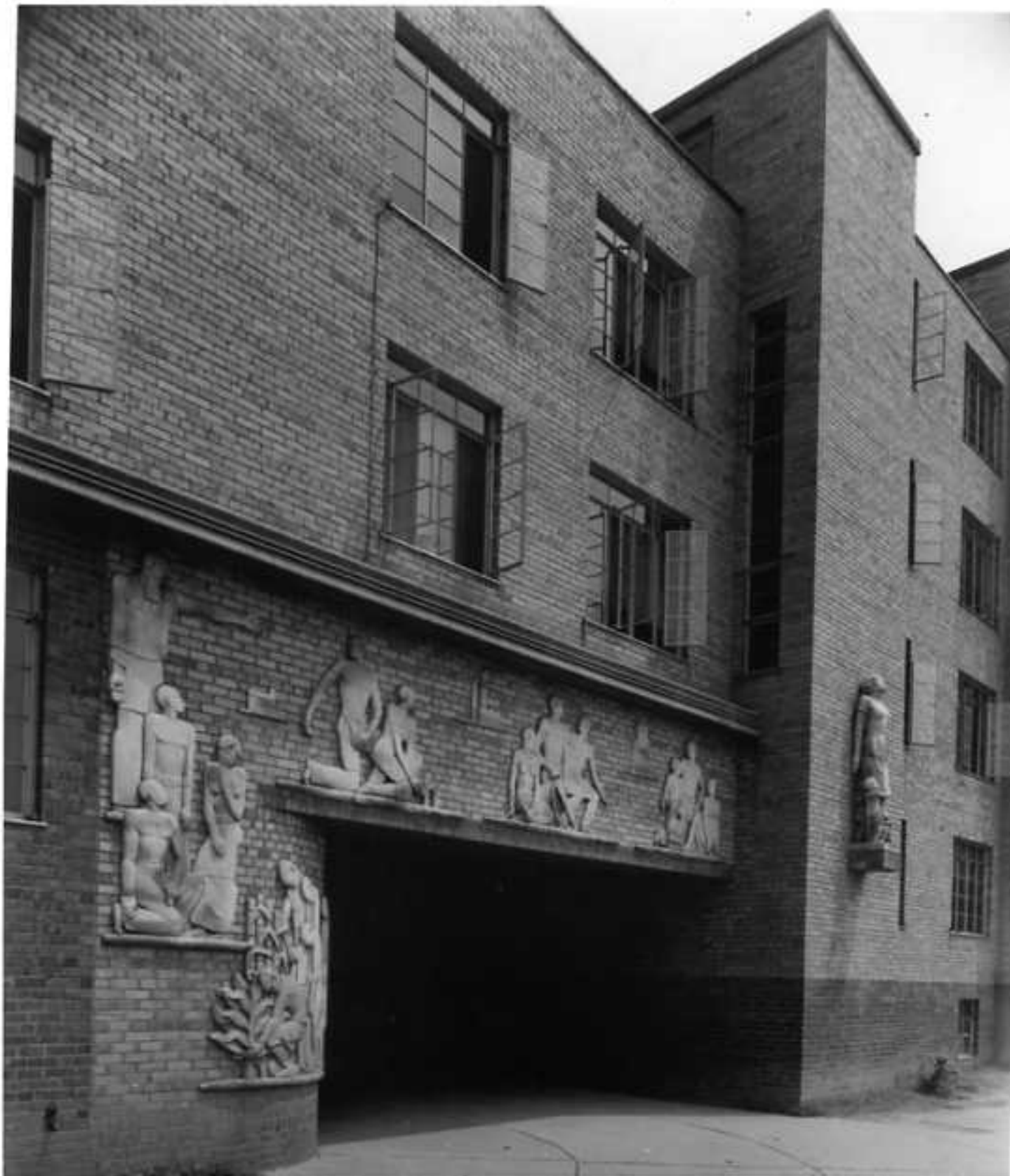
ARCHITECT OF RECORD ROBINSON, PORTER and WILLIAMS DESIGNER Hilyard R. Robinson PROJECT LANGSTON TERRACE DWELLINGS (Archway showing symbolic sculpture) DATE 1937 AUTHORSHIP: Solely Responsible for Design
