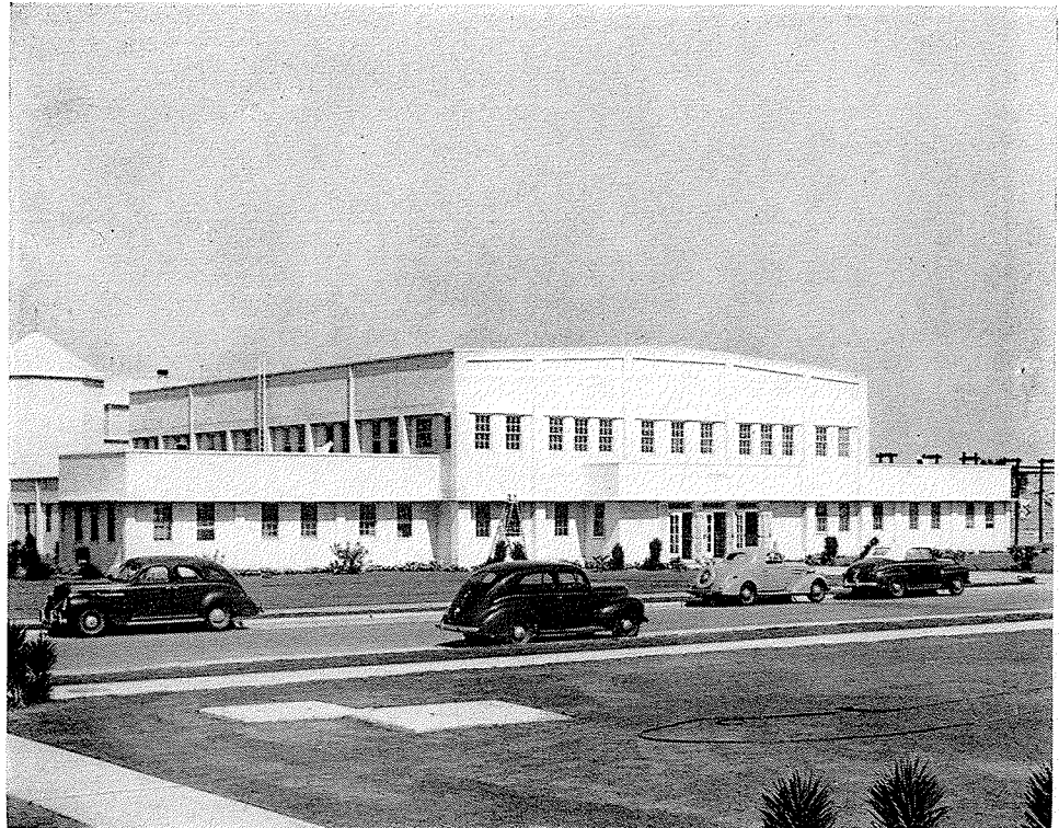
Gymnasium - U. S. Naval Facility in South East
