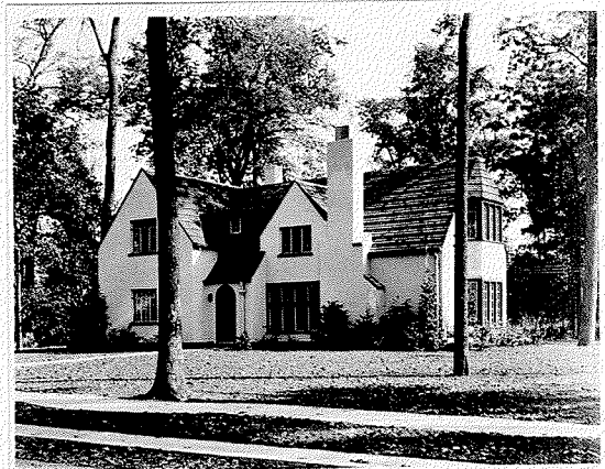
RESIDENCE, BLOOMFIELD HILLS, MICH. STREET ELEVATION 8 ROOMS - COST $22,000.00 OWNER - DR. EUGENE SMITH, JR.
