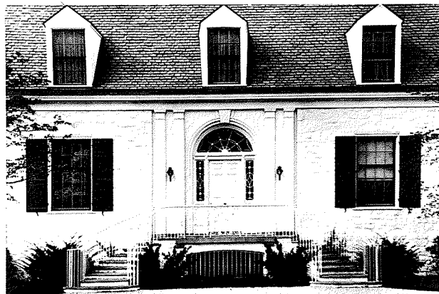
MAIN ENTRANCE OF RESIDENCE AT GREENWICH, CONN. FOR RICHARD I. ROBINSON, ESQ. 140,000 CU. FT. $126,180.00
