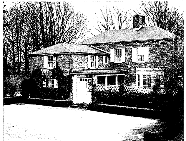
ENTRANCE VIEW OF RESIDENCE AT NEWPORT, R.I. FOR FRANCIS TAYLOR, ESQ. 55,000 CU. FT. $25,000.00
